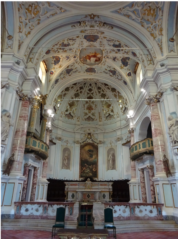
Abb. 4. Church of Saint Antonio in Villa Pasquali. Seismic improvements works, repair and conservation works have just been completed. Foto: Soprintendenza Archeologia, Belle Arti e Paesaggio per le province di Cremona, Lodi e Mantova.
